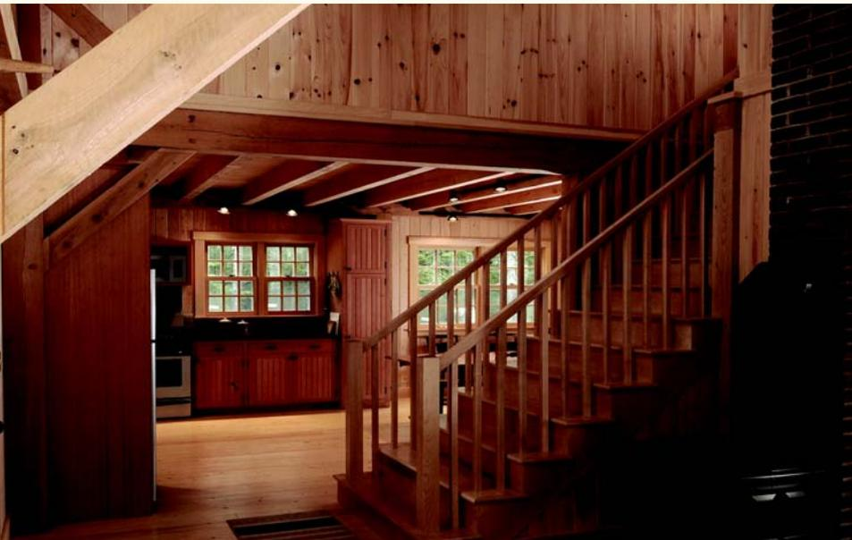
Beauty and character of traditional timber frame homes are a result of natural materials being crafted by the hands of the builder. Each building frame is a unique wooden sculpture composed of large wooden beams that lock together with wooden pegs to form the visible interior.
